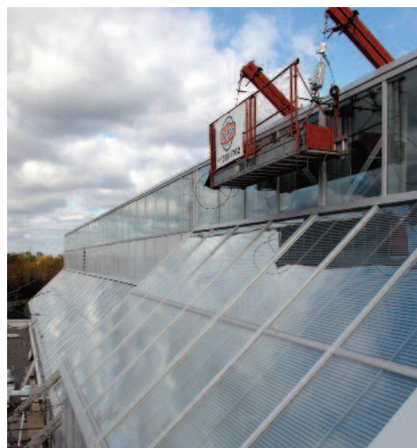
Vision Control® exterior application at a building site in Quebec, Canada
